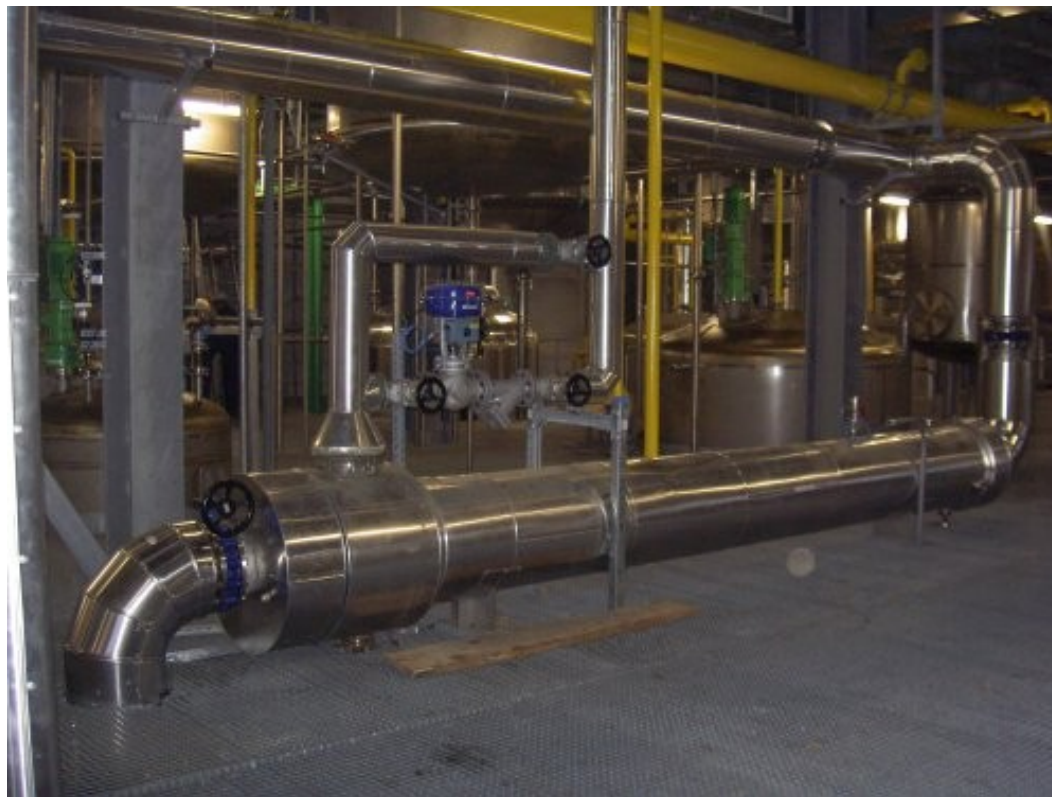
Methanol Recovery Reboiler 2005, Poland
